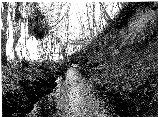
Fig. 2. Asymmetrical slope form of the Tamagawa Josui Canal. Sunny cliff is south-facing left bank and slope in shadow is north-facing right bank.
