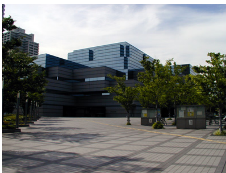
Osaka Prefectural Central Library
