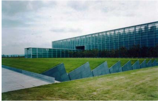
<<Kansai-kan appearance (northwest view)>>
