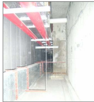
<< Underground stacks (Double wall for waterproofing)>>
