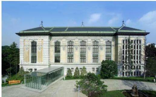
<<ILCL frontage (east view)>>
