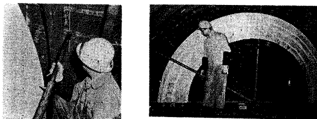
Fig.31 Measuring circularity of inner hull cylinder by using special measuring apparatus.
