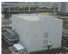
Fig. 1 View of New Climate Testing Laboratory
