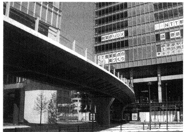
Photo 1 Pedestrian Bridge after Construction is Completed
