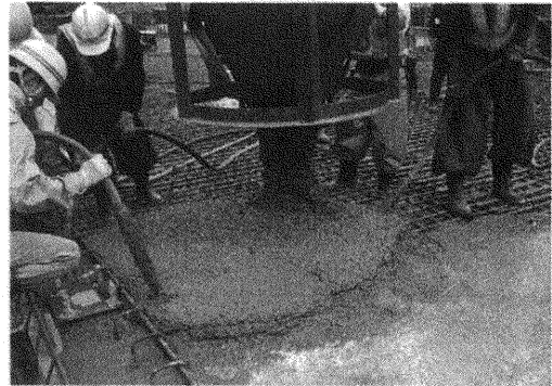
Photo 3 Placing Situation (Vibratory Compaction Type)
