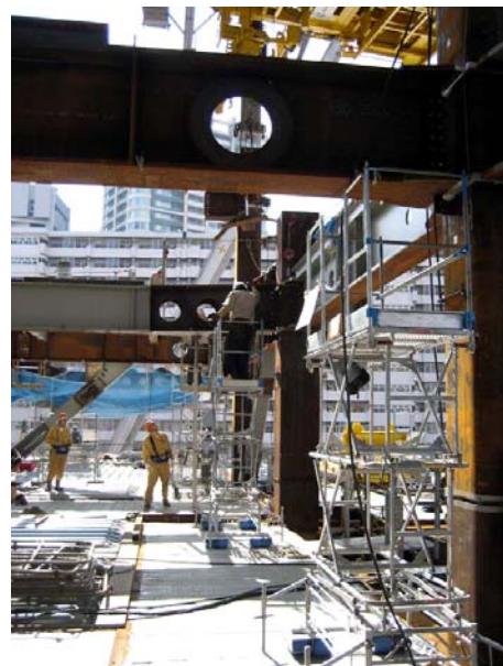
Photo 1 鉄骨工事用足場 Special Rolling Tower for Steel Frame Work
