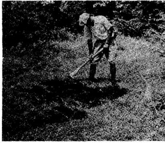
写真-3.8 積苗工に使う切芝の現地採取<sup>7)</sup>
