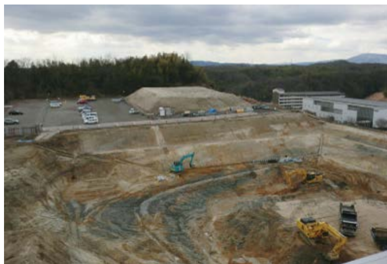
Digging started in Nov. 2016 (Feb. 13, 2017)
