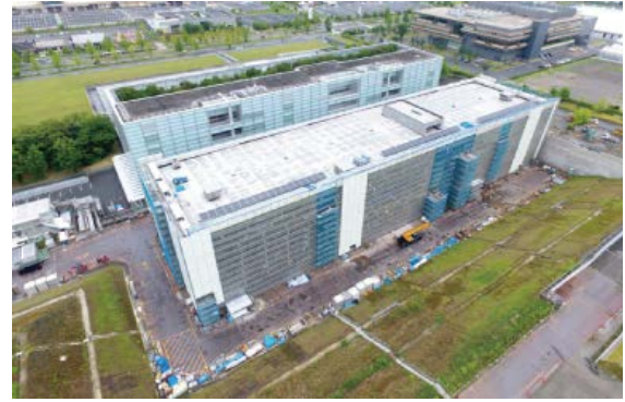
Exterior wall construction (July 26, 2019)
