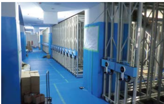
Placement of shelves (May 24, 2019)
