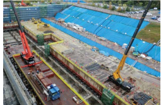
Working platforms constructed by cranes (Oct. 17, 2017)
