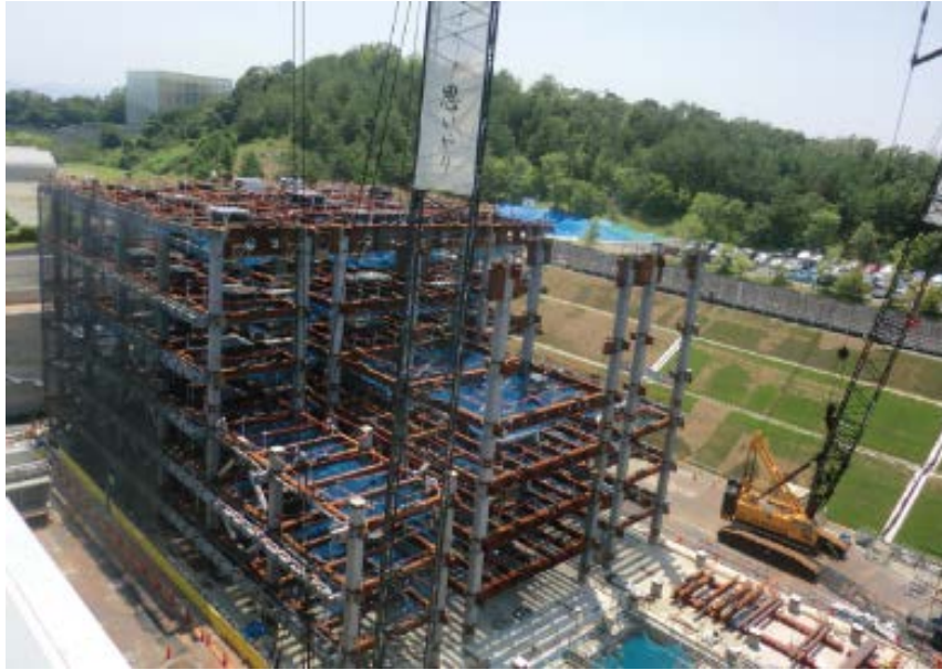
Finally, steel columns start to appear! (June 25, 2018)
