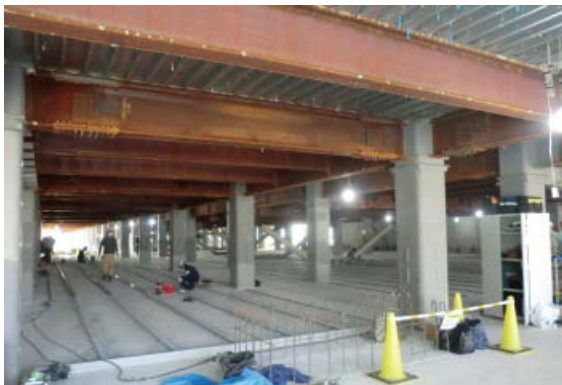
Interior work began. Placing rails for compact shelves (Oct. 26, 2018)
