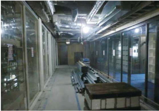
Construction of corridors for unobstructed view of stacks (Sep. 27, 2019)
