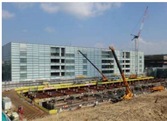
Construction site seen from the south (Feb. 26, 2018)
