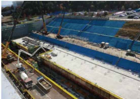
Concrete placement on the first basement floor (Nov. 27, 2017)
