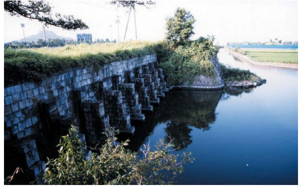
Figure 3-13. Land-reclamation-related Remains of the Yatsushiro Seacoast (Yatsushiro City, Kumamoto Prefecture)
