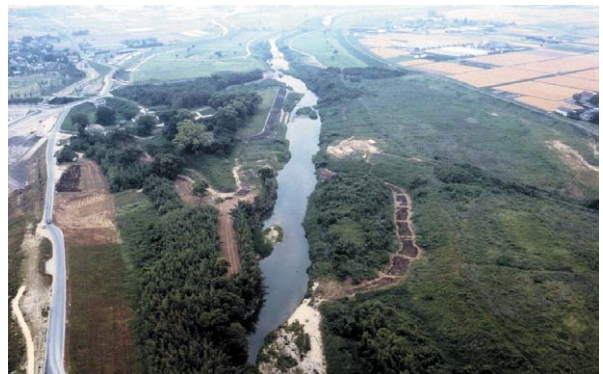
Figure 3-17. “Ishiibi” Dam and the River Tabuse (Saga City and Yamato-cho, Saga Prefecture)
