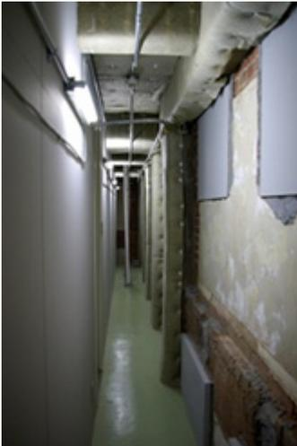
Photo 8: Boarded windows (right), buffer corridor (center) and wall of stacks (left)
