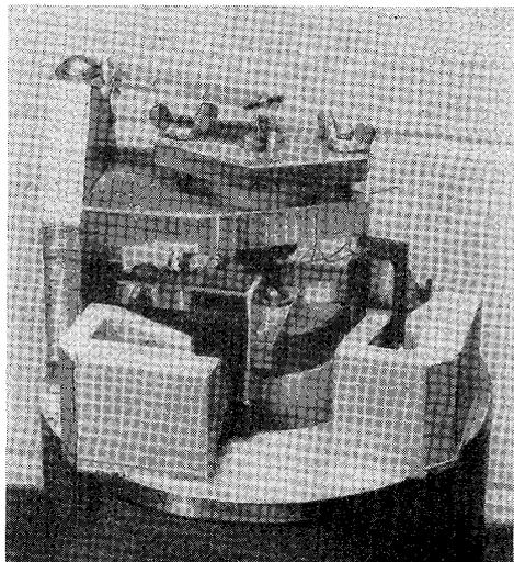
Photo. 1. Driver-pickup system of the resonant column device
