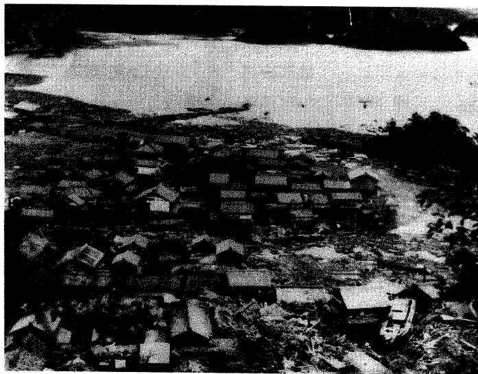
Fig.18 View of Asakawa village crushed or washed away by the 1946 Nankai Tsunami: Some houses at Sugasaki district in the center of the photograph were protected from the attack of the tsunami by the Torigoe groin and a small island on the right hand side of this picture. Many houses at Higashi districts were destroyed by stray ships.
