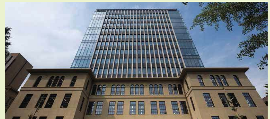
The Promotion and Mutual Aid Corporation for Private Schools of Japan / General Facility Expenses / Building 3, Waseda University / Shinjuku-ku, Tokyo
