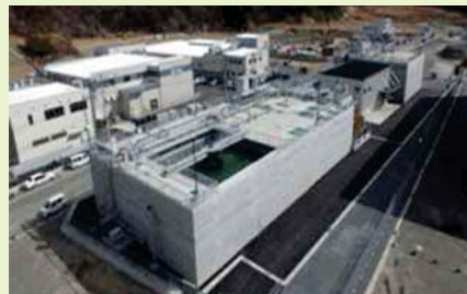
Private Finance Initiative Promotion Corporation of Japan / Improvement Project of Wastewater Treatment Facility in Seafood Products Processing Centers / Wastewater Treatment Facility / Onagawa Town, Miyagi Prefecture
