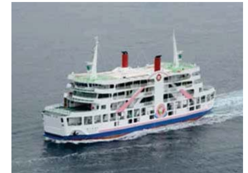
Japan Railway Construction, Transport and Technology Agency / Sakura Fairy / Dai-ni Sakurajima Maru / Kagoshima City, Kagoshima Prefecture
