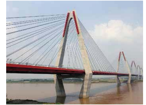
Japan International Cooperation Agency / Nhat Tan Bridge (Vietnam-Japan Friendship Bridge) Construction Project / Nhat Tan Bridge / Hanoi City, Vietnam
