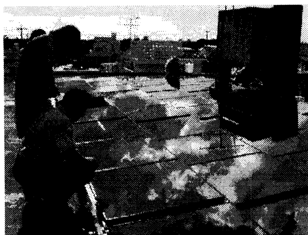
Figure 2 Setting of thermo-couples around PV modules on the rooftop of the experimental house.
