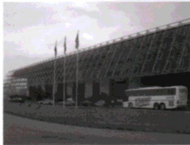
Rio Centro convention Center
