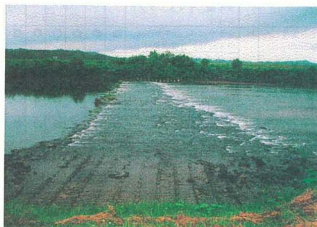
写真-1.2 No. 1地点床止め
