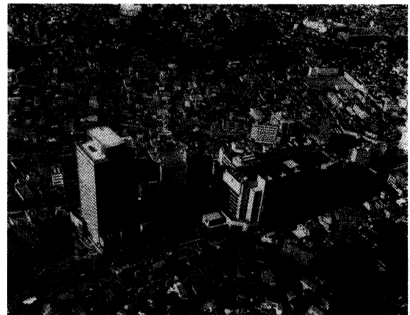
Photo 1 Complete View of this Building
