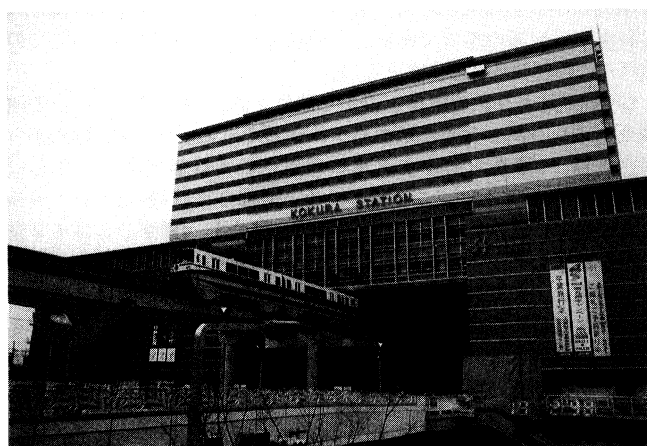
Photo 3 Front View of Station
