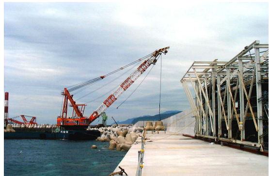
Photo 2 護岸施工状況 (Construction of Seawall)
