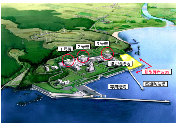
Fig. 1 泊原子力発電所3号機完成図 (Finished view of the Tomari nuclear power station unit 3)
