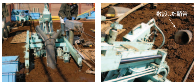
図18 鞘管引き込み拡張推進の状況と敷設した鞘管 Fig. 18 Sheath pipe in boring, propulsion, and laid conditions.
