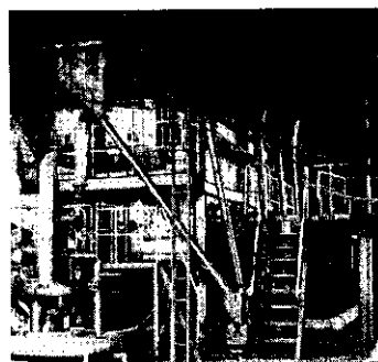
Photo. 1 Firing zone of 1,000 t/day-furnace
