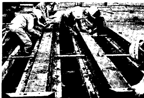
Photo.2 Placing of expansive concrete
