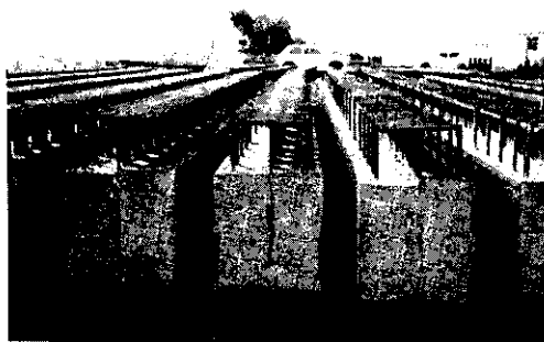
Photo.3 Precasted H beam
