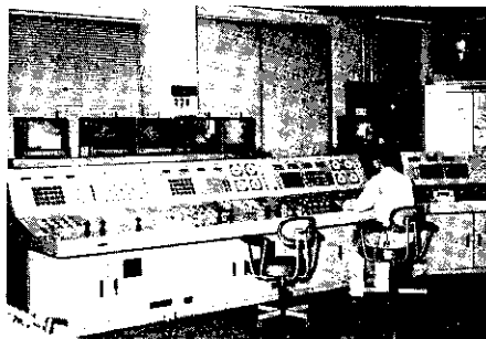
Photo. 2 Operation room of reclaiming machine
