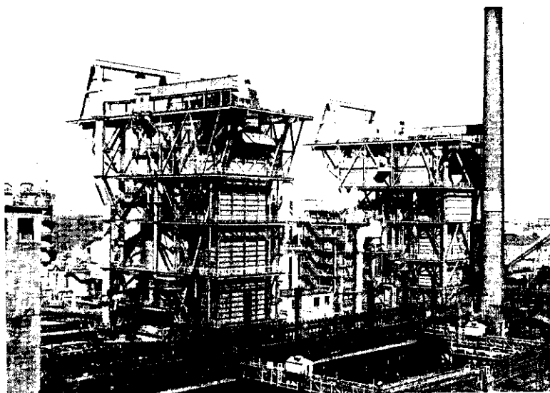
Photo. 1 General view of No. 2 CDQ
