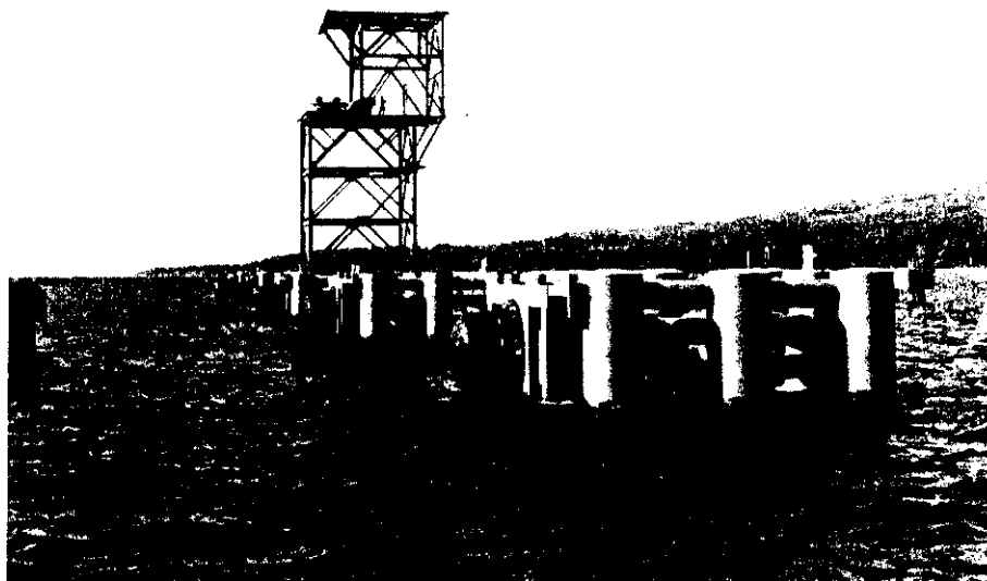
Photo. 2 Dolomite loading facilities at Alcoy site
