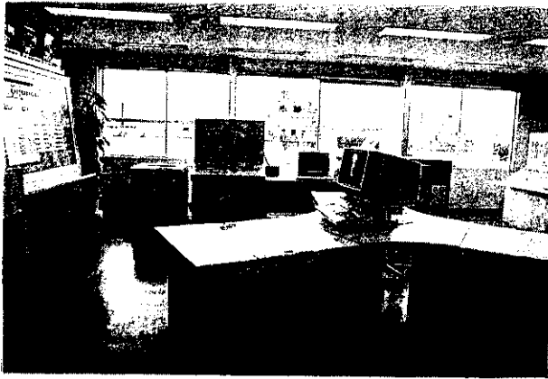
Photo 1 View of control room
