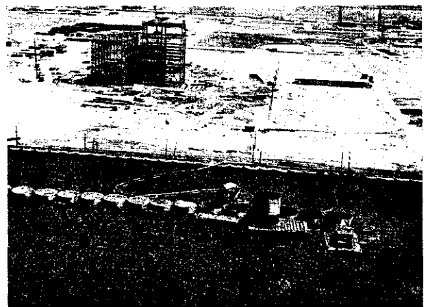
Photo 5 Prefabricated corrugated cell bulkhead method at Mizushima Works
