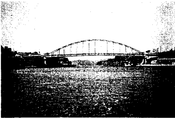
Photo 1 View of Oku-Nagashima bridge
