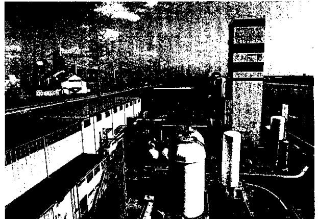
Photo 1 General view of No. 12 oxygen plant
