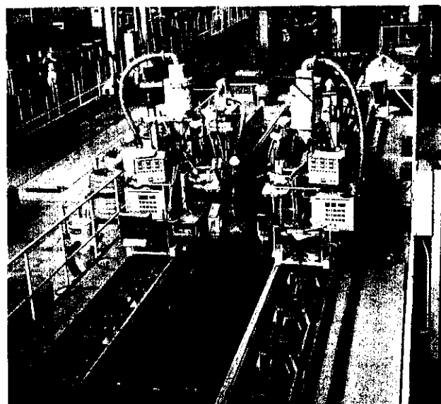
Photo 3 3-electrodes SAW (3KX) apparatus for corner seam welding
