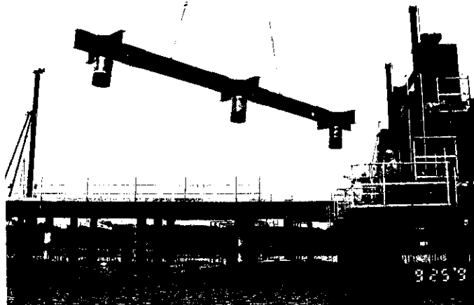
Photo 6 Installation of prefabricated pile heads by STEP method
