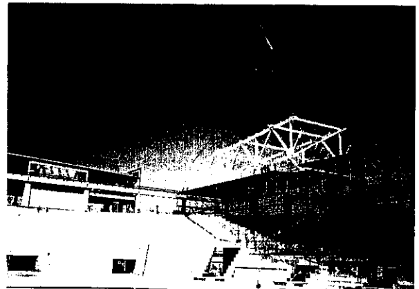
Photo 3 Hoisting boxed truss
