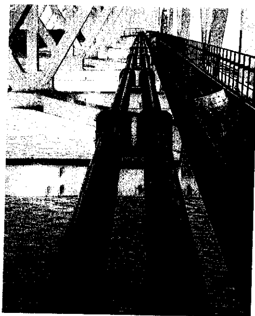
Photo 16 Water pipeline on Akashi Kaikyo Ohashi Bridge
