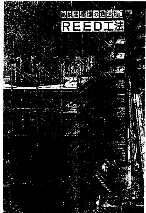
Photo 21 Composite pier (REED method)
