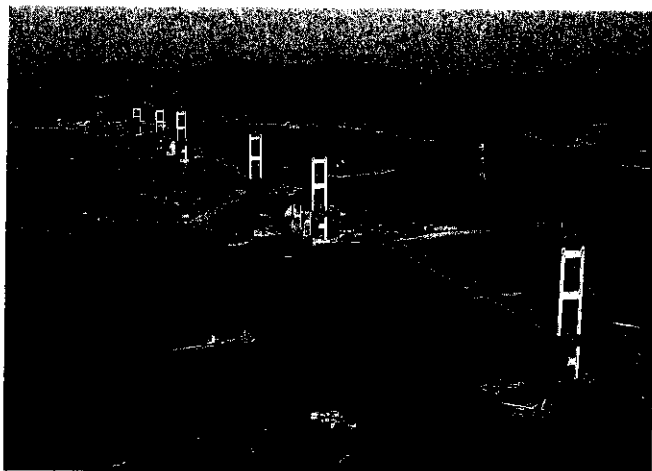
Photo 8 Kurushima Kaikyo Bridge
