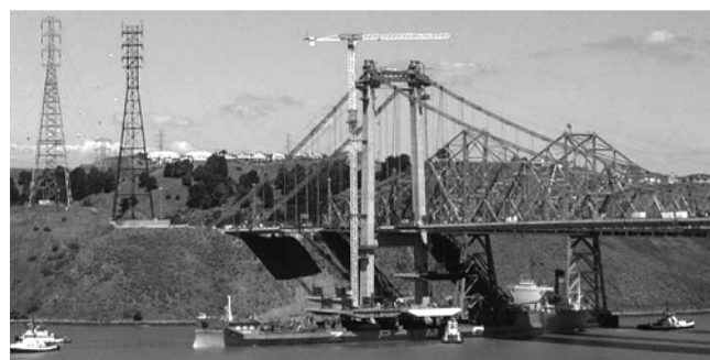
第 12 図 係留解除状況 Fig. 12 Releasing of anchor lines with tug boats
