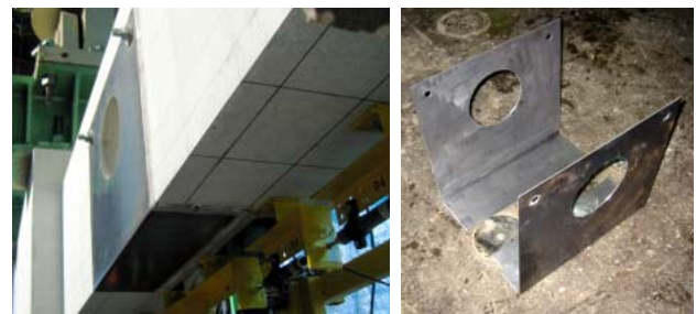
Photo 1 補強状況 View of Strengthening Portion
