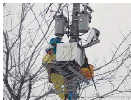
Fig. 6 Camera observation device for lightning strikes
