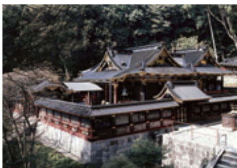
National Treasure Kunozan Toshogu Shrine Honden main hall, Ishi-no-ma hall and haiden altar (Shizuoka City, Shizuoka Pref.)
