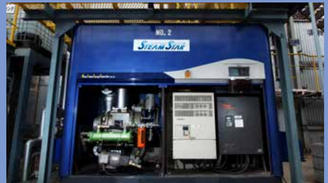
Kobe Steel, Ltd. developed a small-scale steam heat electric generator. Developed as part of a NEDO project that focused on utilizing steam efficiently without wasting pressurized energy. Achieves high-efficiency electric generation with steam as the heat source through a small-scale once-through boiler which was deemed hard to achieve in the past.
