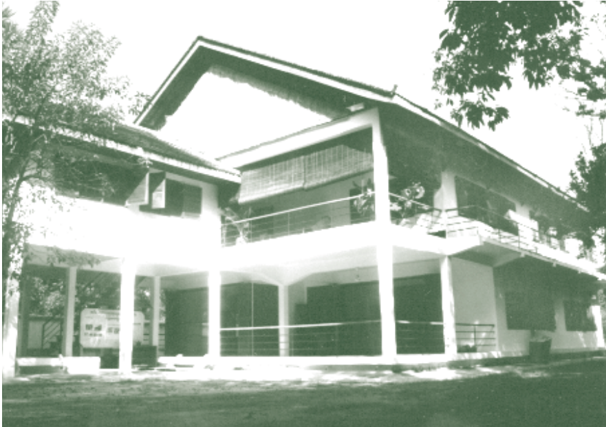
The Sophia House, built in 1996, facilitates the training of local preservation specialists in Cambodia.
