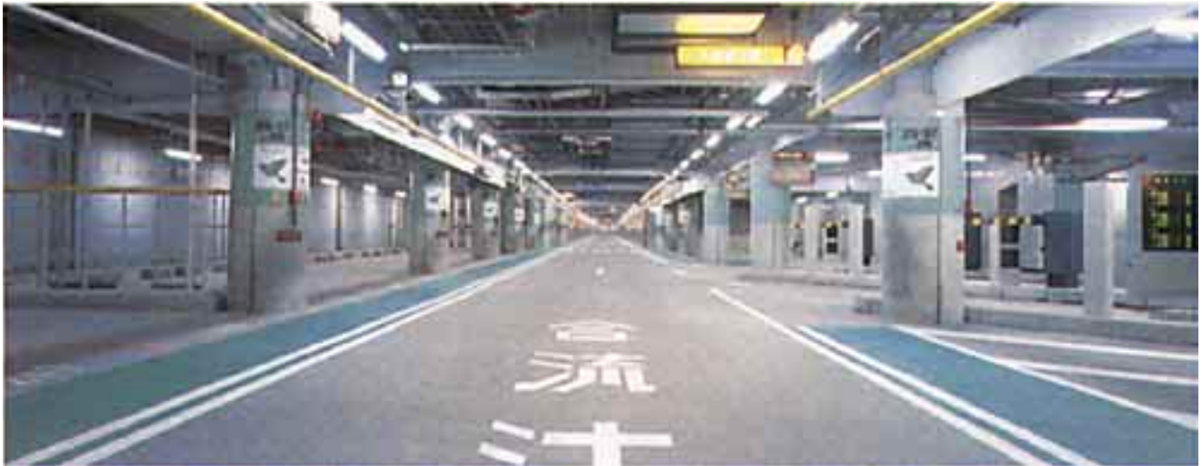
Photo 5 Parking Lot (2nd basement floor)
