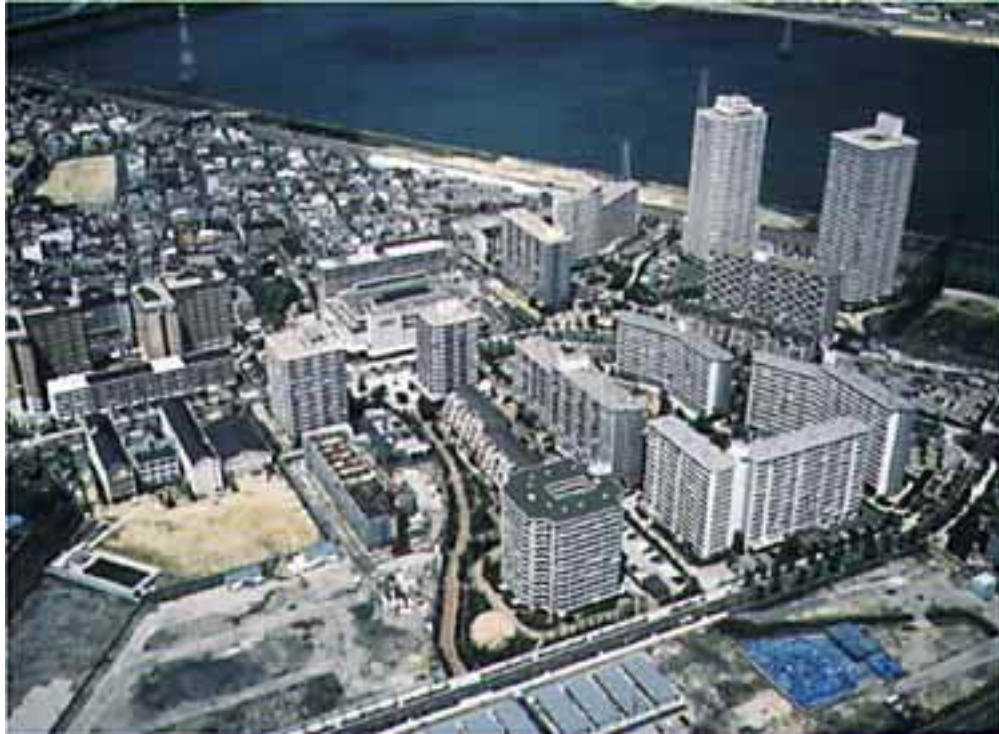
Photo 2 Work Progress in Takami District
