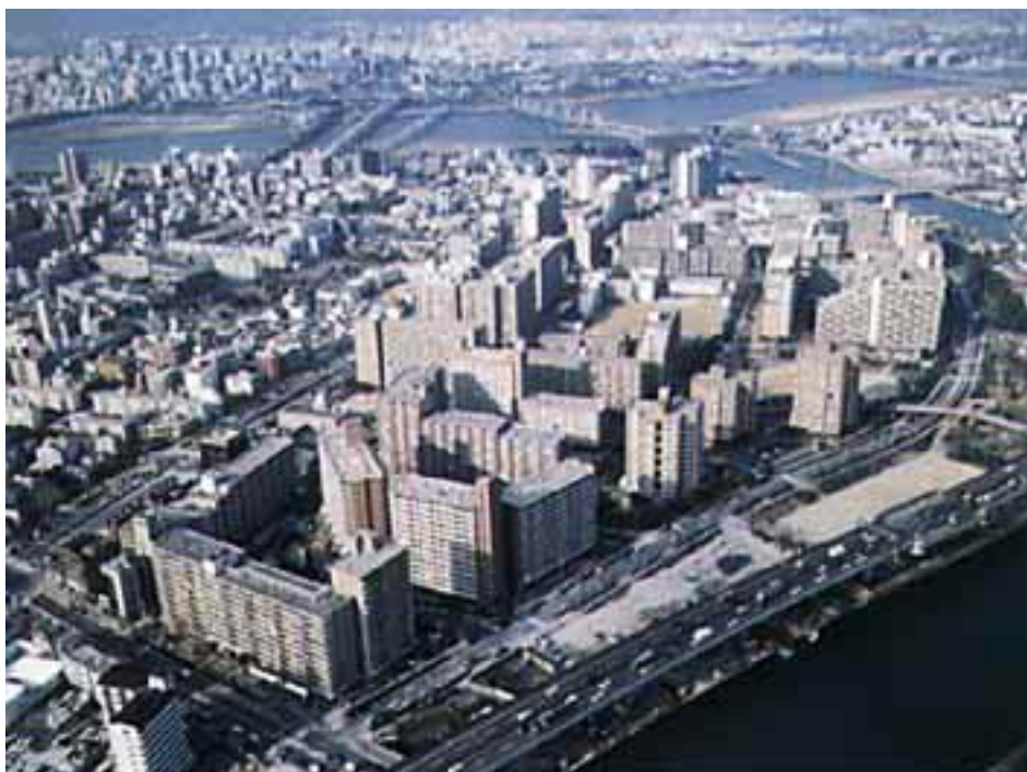
Photo 1 Work Progress in Yodogawa Riverside District
