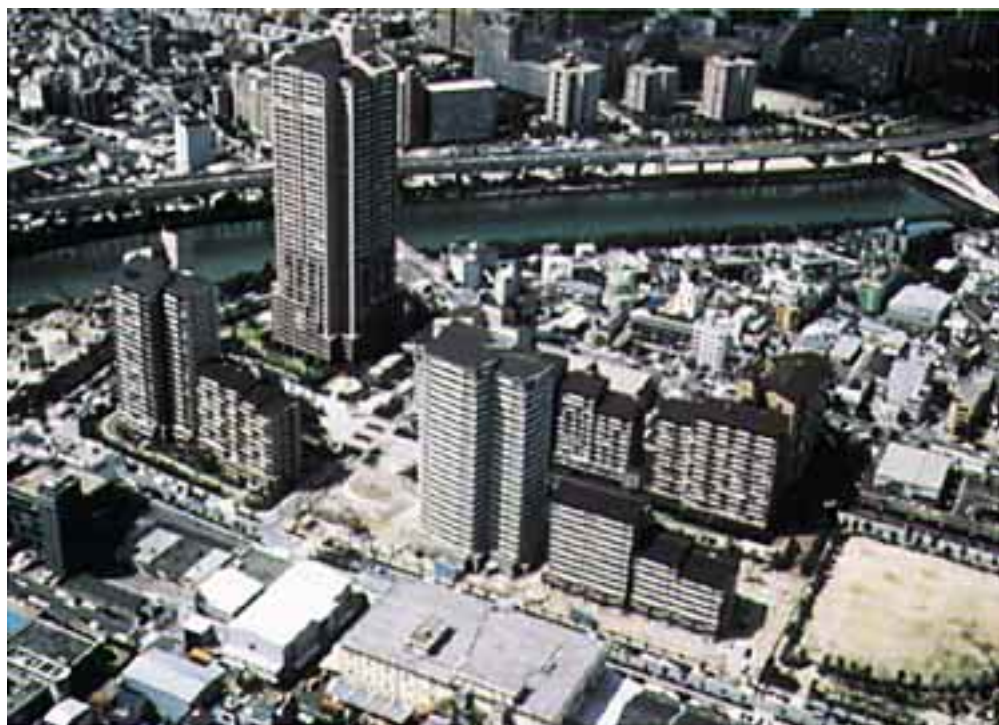
Photo 3 Work Progress in Sakuranomiya-nakano District
